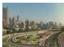
MUMBAI COASTAL ROAD MEGA PROJECT
