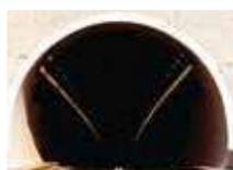
AIROLI-KATAI NAKA TUNNEL
