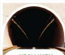
AIROLI-KATAI NAKA TUNNEL
